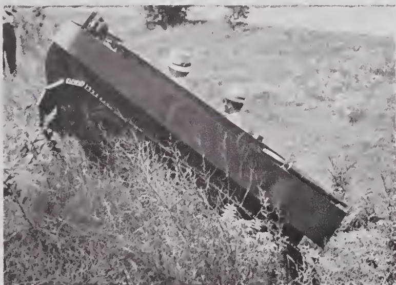
FIGURE 28. Pilot model of T-15 Weasel negotiating 25-degree grade on dry turf.
